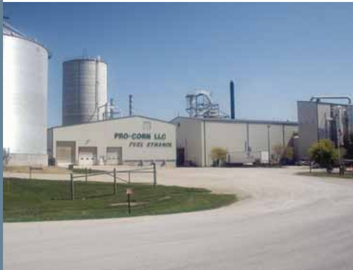
The Pro-Corn Ethanol Plant in Minnesota
