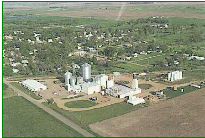
Broin Enterprises Ethanol Plant Scotland South Dakota
