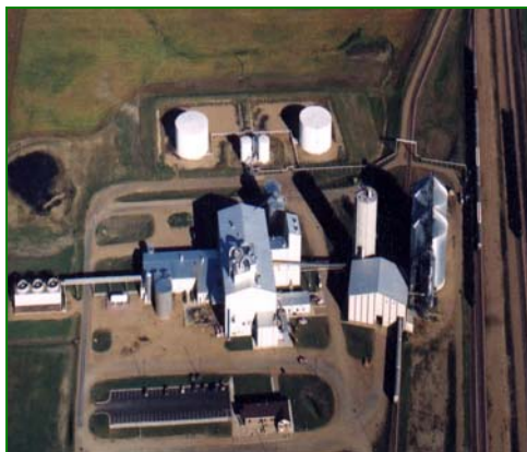
Great Plains Ethanol Plant Chancellor South Dakota
