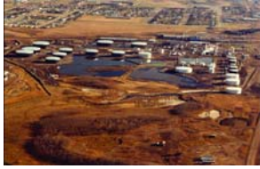
Lloydminster Ethanol Plant
